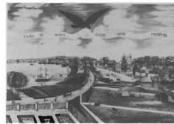
Figure 16 – Depiction of New Orleans as seen from the Marigny Plantation, 1803. Courtesy of Chicago Historical Society.
