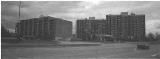
4 The fulfillment of the promise of the Hochhausstadt: "Hilberseimer's barren, gloomy, menacing drawings prophesy a city without streets, even worse, if that's possible, than that which has actually been realized." 3
