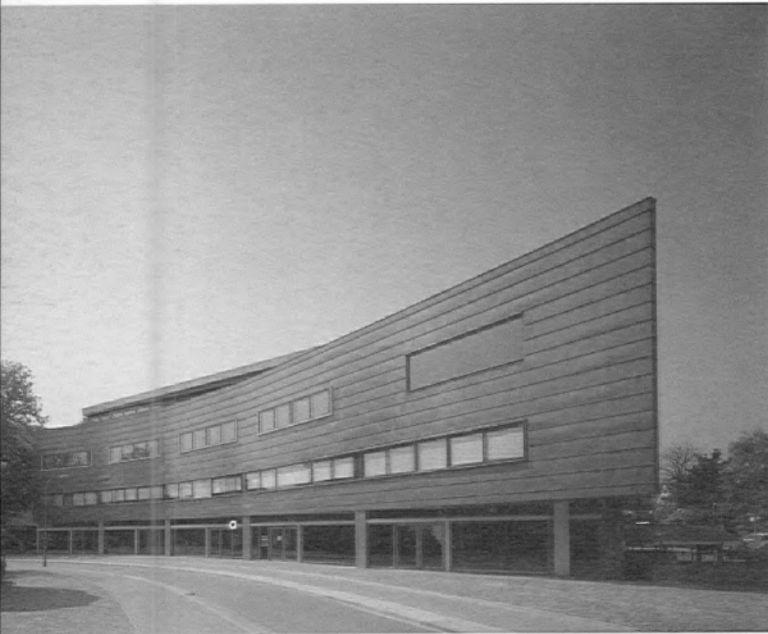
Multi-functional Building, Hilversum
