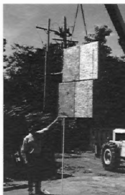
Mock-up Assembly 1/3 Full Scale
