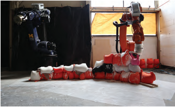
The building process of section 01 by two robots (East and West)
