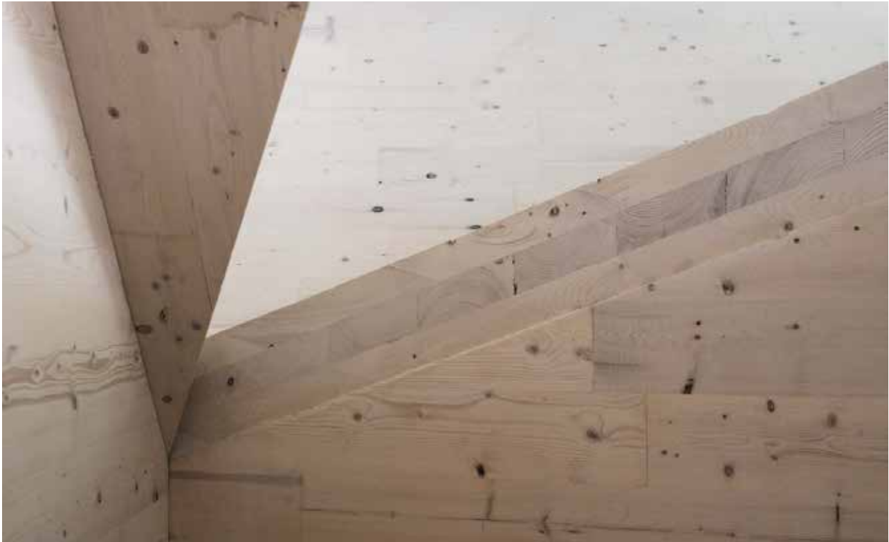
Detail, Four Corners, Ultramoderne, Boston Society of Architects, "Urban Timber," exhibition, 2014
